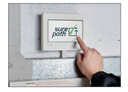
When the screen is active simple touch buttons are also enabled that allow easy access to any fault reports or a password protected engineer's menu.
